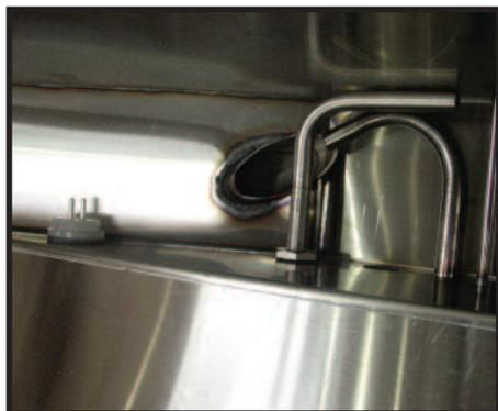
**Sustaining Heater** maintains hot water (140°F) in between racks for the best cleaning results.
